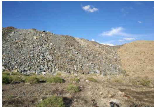
图4-10 废石渣堆ZD23
